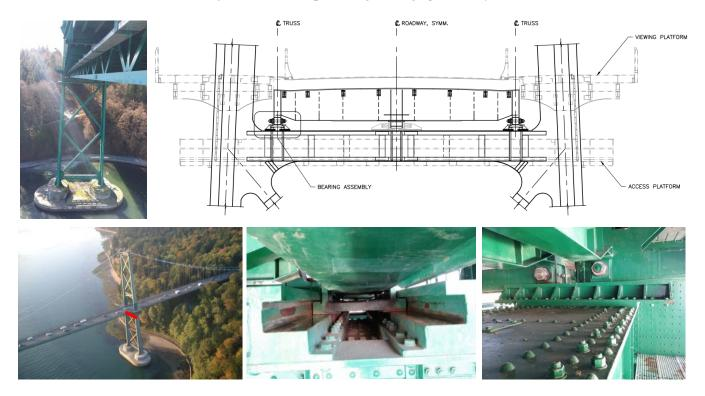
Figure 2. Clockwise from bottom left: Aerial view of south tower with tower strut highlighted in red; view of south tower from below deck; view of tower segment from drawings showing tower strut deck diaphragm, truss bearings; bearings within bearing guides supported on top of tower strut; previous deteriorated bearing shoe within bearing guides.
